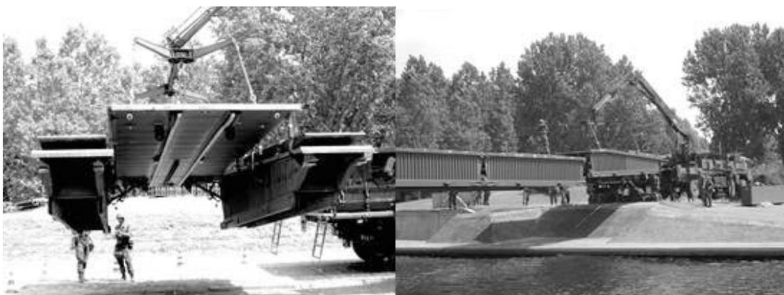
**Fig. 2. Erection of the DoFB bridge; lifting of the drive-on segment and setting of a segment on the launching beam**
