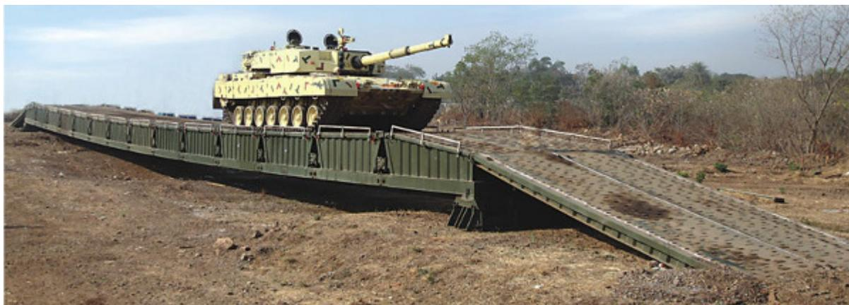
**Fig. 11. View of 46m MLC 70 Modular Bridge [14]**
