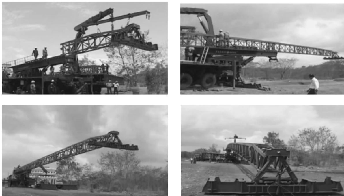
**Fig. 12. Subsequent stages of setting up launching beam of the 46m MLC 70 Modular Bridge [16]**
