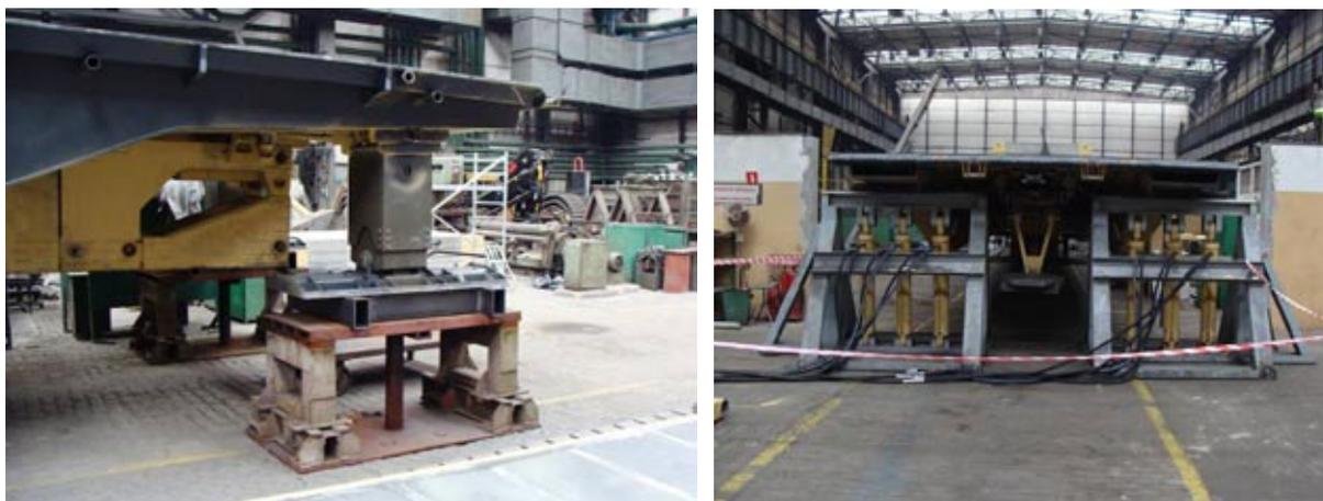
**Fig. 6. Manner of supporting ends of the main span of the bridge**
