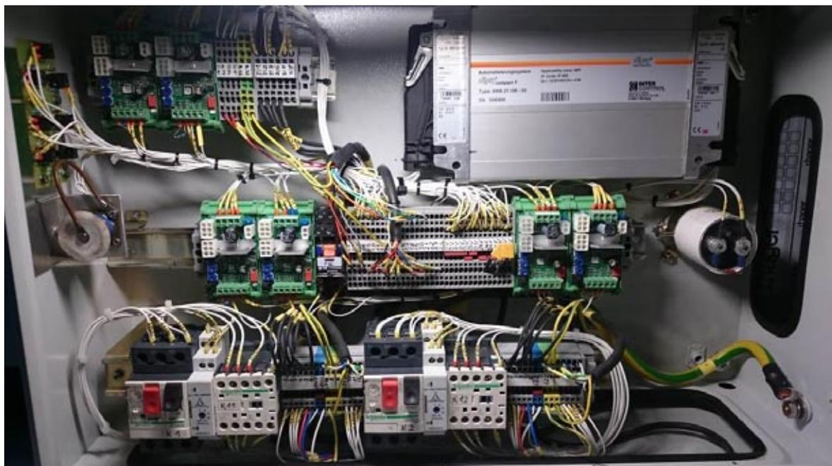
**Fig. 5. Modernized control system installed in the SRK box**
